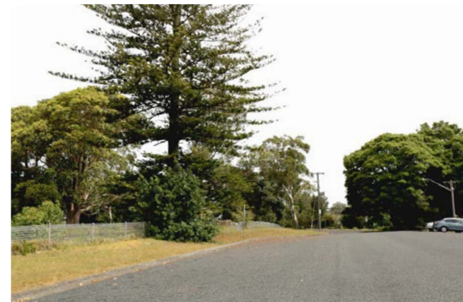
View south along West Street
