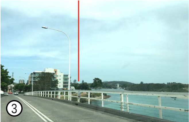
View east along Forster Tuncurry Bridge
